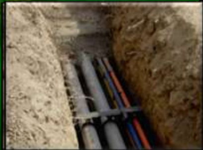
Concrete-Encased Duct Bank
